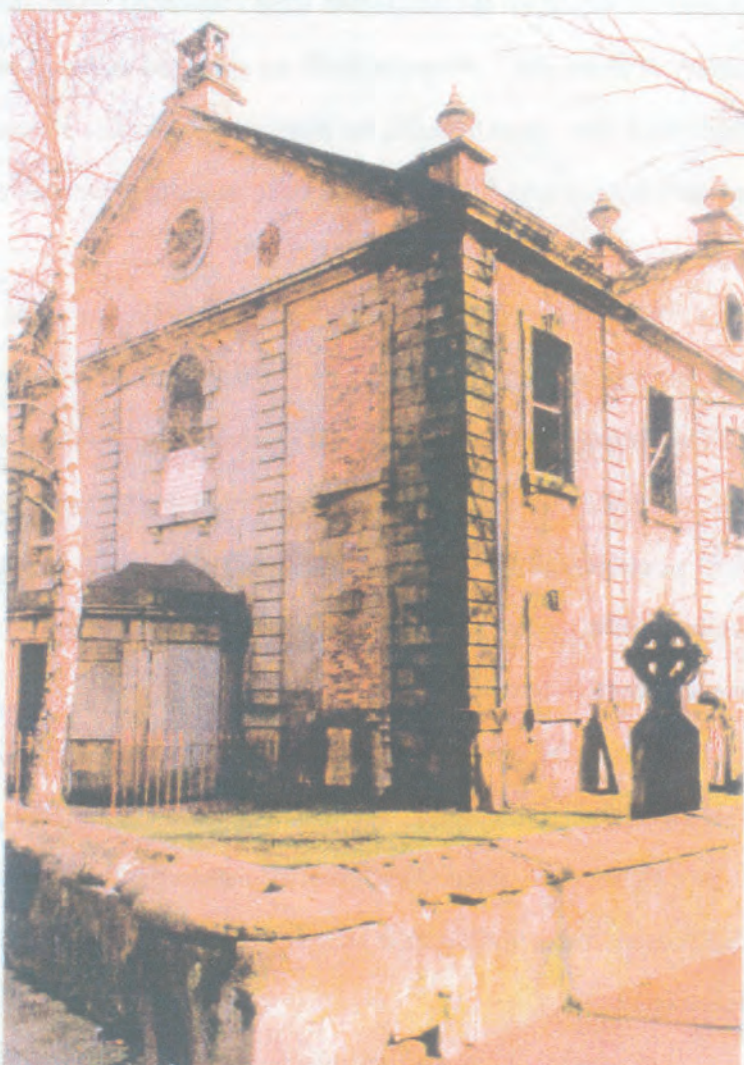
ST. ANDREW'S - BY - THE - GREEN DURING RESTORATION.
